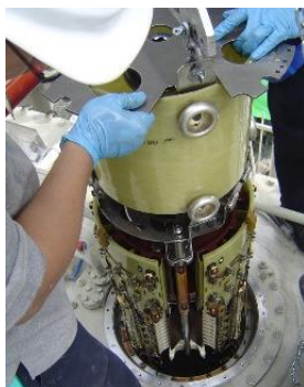
After maintenance, alignment and measurements, the OLTC is being lowered into compartment and put back into operation.
