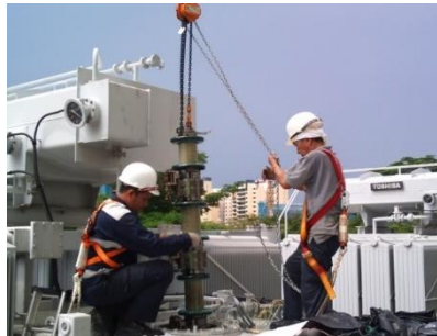
Lifting of the OLTC from the transformer
