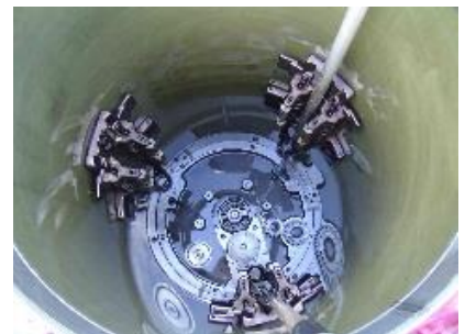
Transformer internal cylinder of OLTC Before and After maintenance.
