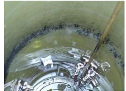
OLTC upon removal from its compartment. Due to long time operation, Transformer insulating cylinder was thickened with carbon residue from breakdown of insulation oil.
