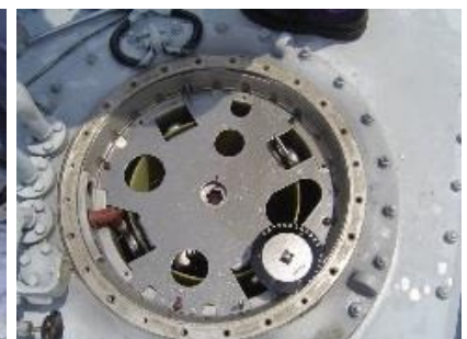
Transformer OLTC Tank Top Before and After maintenance.
