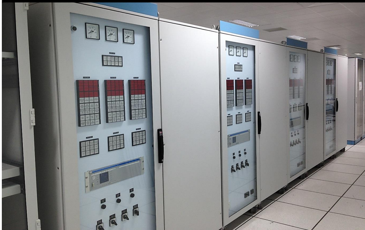
400kV transformer control panel
