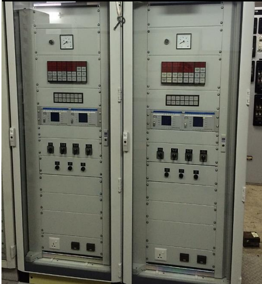
400kV transformer control panel
